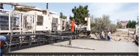
Heavy-duty finishing beams and super smoothers installed in the slipform paving trains are responsible for producing a surface of superior evenness.
